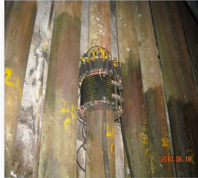
View showing collar placement on one of the Heater Tube.
